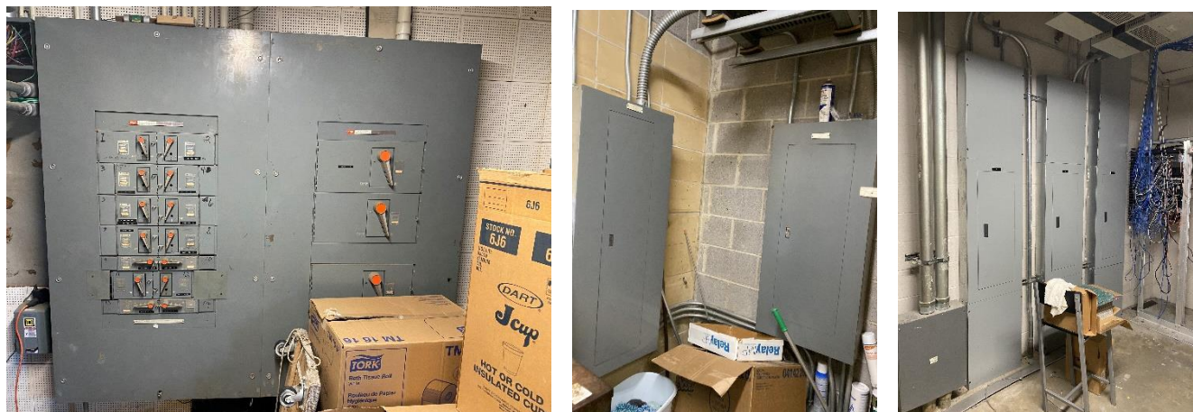
FIGURE 4: NEC EQUIPMENT ACCESS AND WORKING SPACE VIOLATIONS
